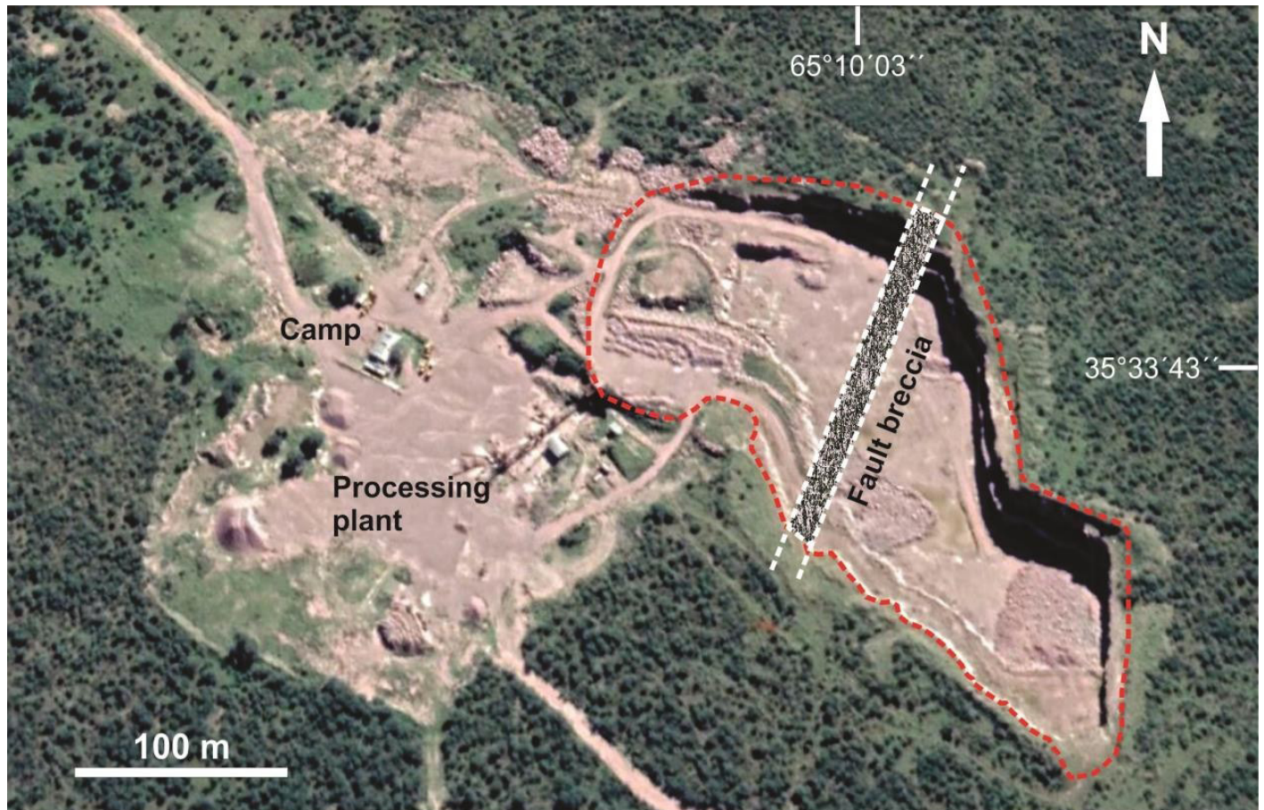
Figure 2. Google Earth satellite image of the Cuatro Pozos sandstone open pit, camp and bulk-rock processing plant (Minería y Servicios S.A.). The original boundary of the sandstone outcrop, prior to mining, is approximately outlined. The actual depth is approximately 21 m. Overburden is a loess-like sediment of variable thickness (up to 1 m) topped with soil, with localized calcrete layers (up to 40 cm thick). The trace of the fault breccia is sketched.
