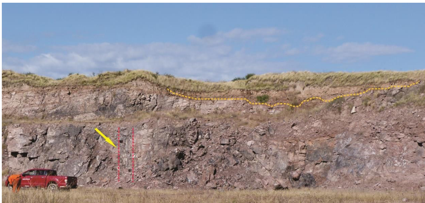
Figure 3. View of the SW margin of the quarry. The wavy dotted (yellow) line shows the contact between the arkose and overlying regolith and loess-like sediments and soil cover. Black stains are Mn oxides that roughly delineate the SW edge of the fault breccia zone; however, the image view is oblique to the strike of the fault zone/breccia, hence what is shown is the width along the bench and not the thickness of the brecciated-mineralized lineament which is 5 to 10 m. The arrow points at a breccia body (between red-dashed lines) shown in detail in figure 5.
