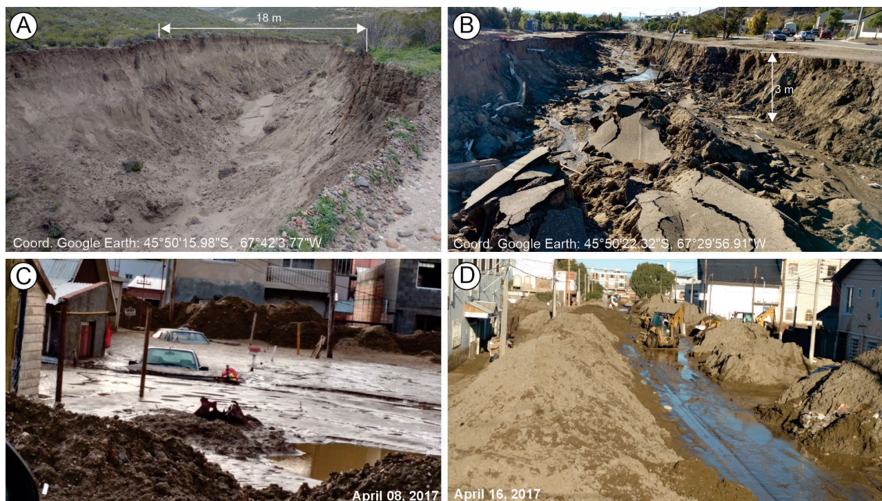
Figure 4. Erosional and depositional features associated with the March–April 2017 extreme rainfall event. (A) V-shaped gullies developed close to the headwaters in the De la Quinta basin. (B) Formation of deep gullies in steep urban areas. Fray Luis Beltrán Avenue, Km. 3 drainage catchment. (C–D) Sediment deposition in lowland areas of the (C) Laprida sub-basin and (D) De La Quinta catchment (location in Fig. 1B).
